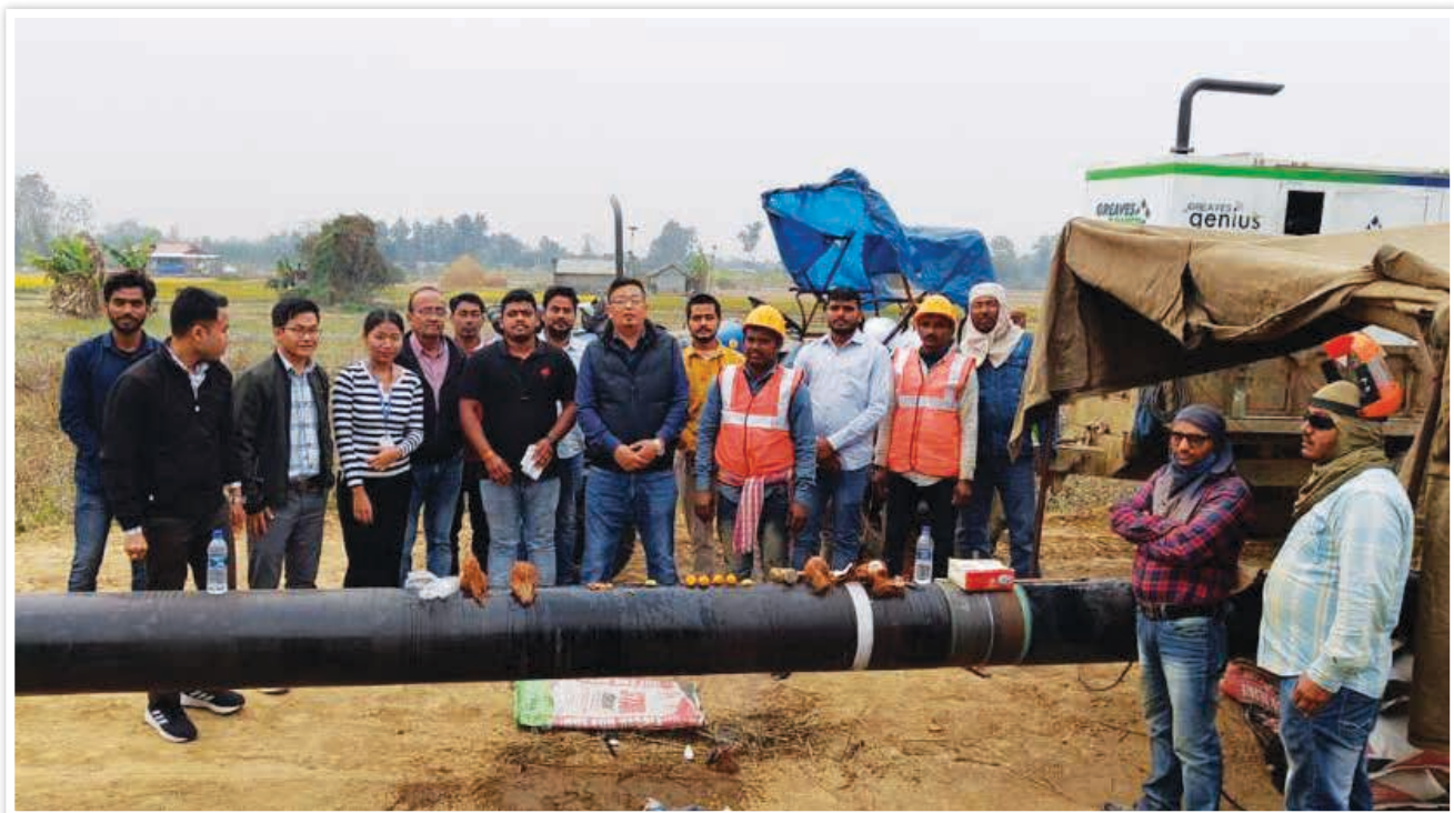
Construction activities for the Dimapur-Kohima-Imphal section commenced on 11.02.2023
