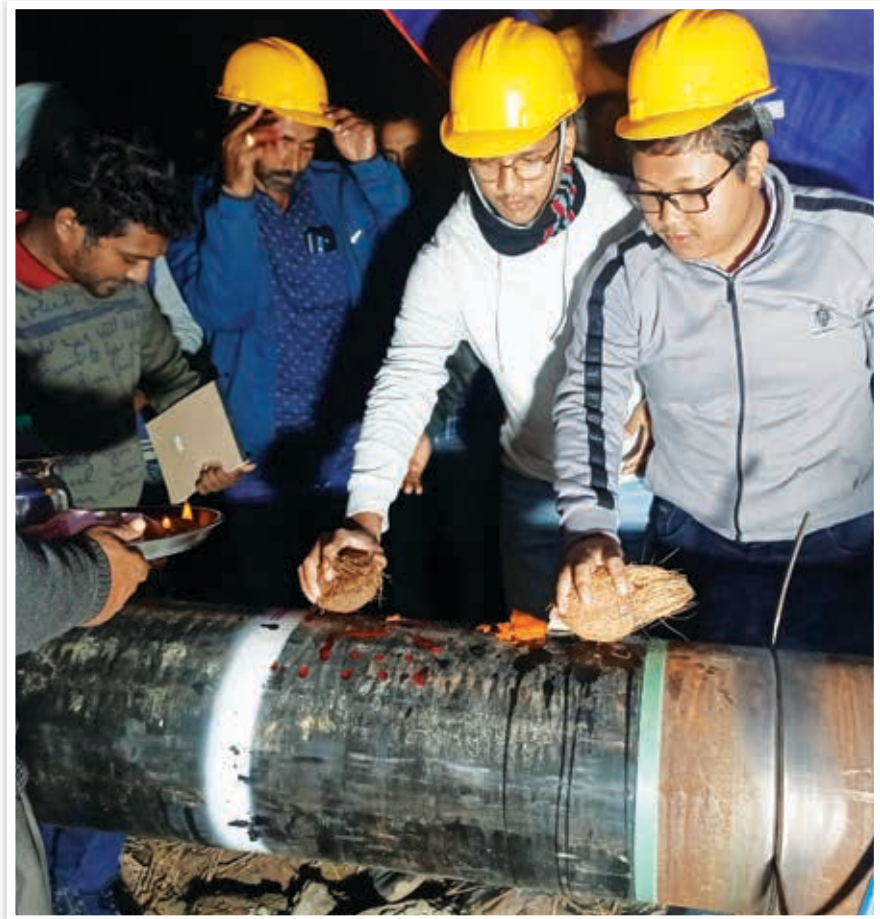
Construction commenced for the Panisagar-Aizawl pipeline in Tripura on 06.01.2023
