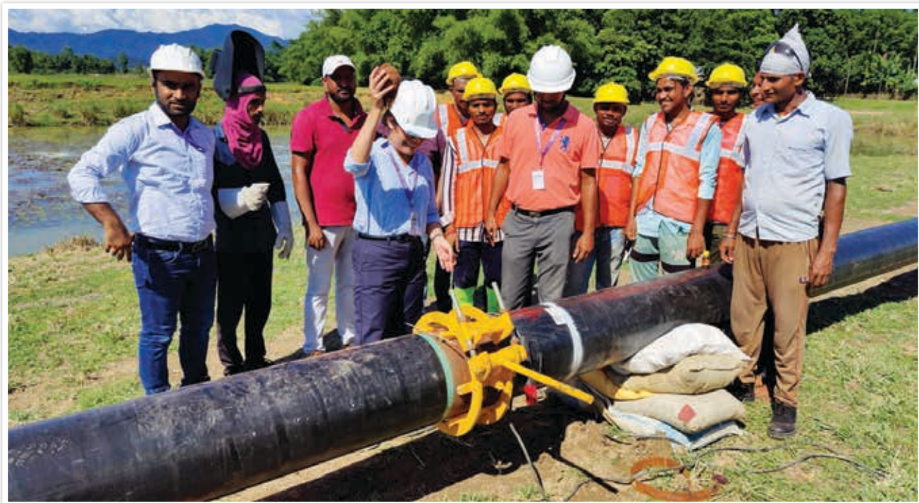
Construction of the Banaskandi Feeder line commenced on 07.09.2022
