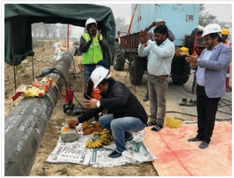
Construction commenced for the Siliguri-Gangtok pipeline in West Bengal on 16.01.2023
