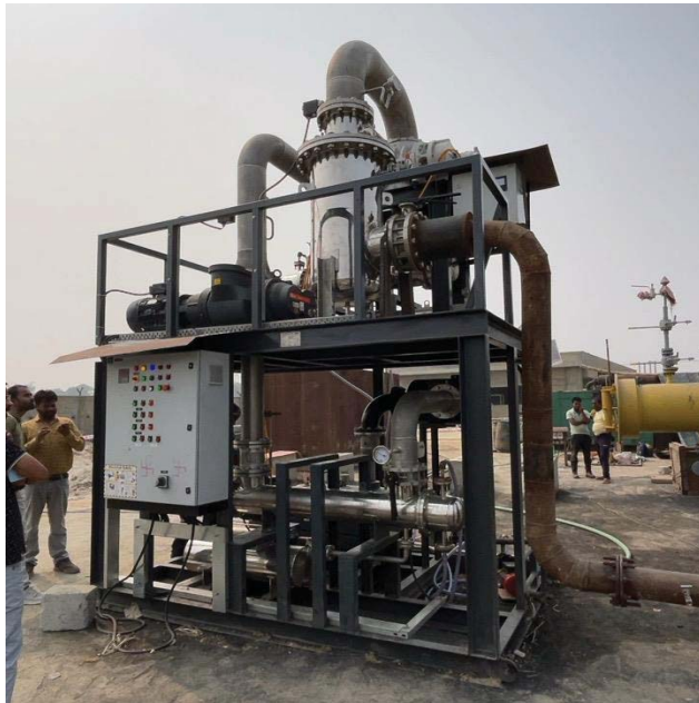
Vacuum cleaning in progress in the Guwahati-Numaligarh pipeline.
