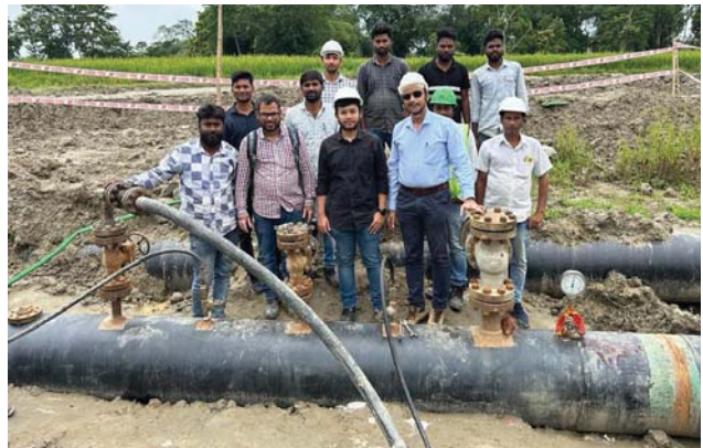
Welding, Lowering and Hydrotest of Guwahati-Numaligarh mainline have been completed.
