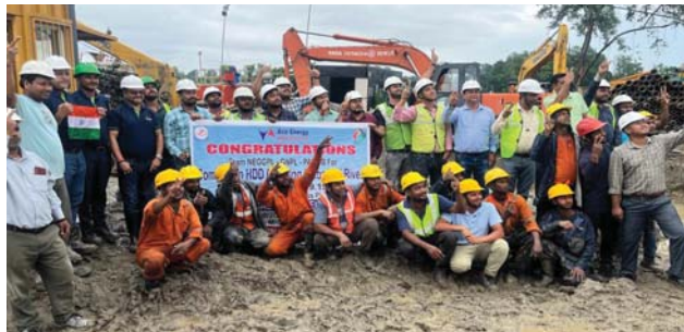
HDD pulling in Subansiri river having a length of 3.5 Km in Spread C of the Guwahati-Numaligarh pipeline successfully completed on 17.06.2023.
