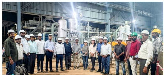
Start of compressor Mechanical Run Test (MRT) at Baihata Compressor Station on 12 November 2025
