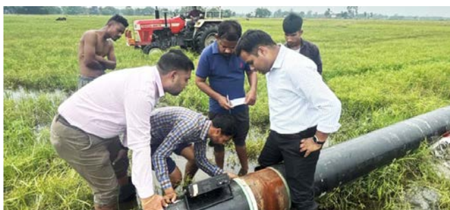
Pipeline works being carried out through highly disputed plains along Siliguri-Gangtok Pipeline Section
