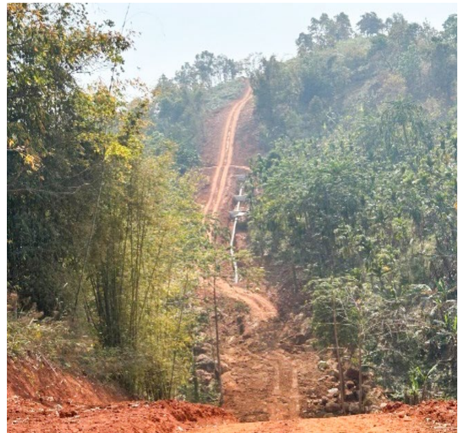
Pipeline works being carried out at tough terrains along Guwahati-Silchar Pipeline Section
