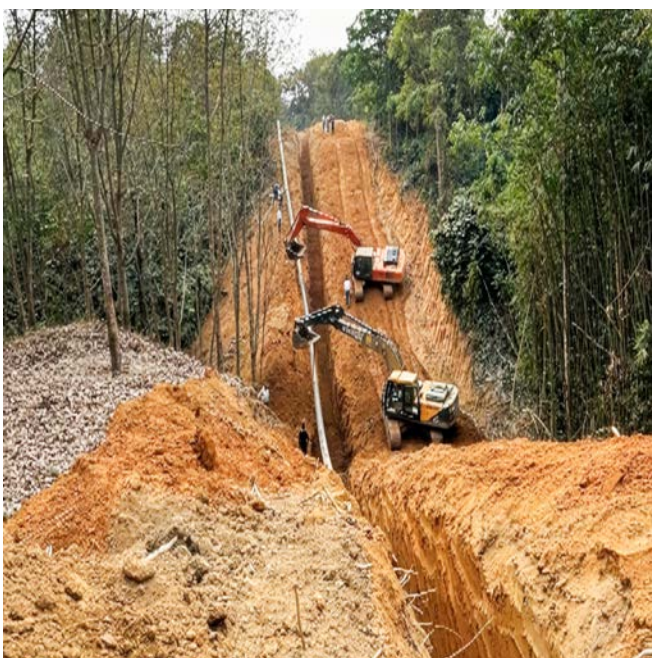
The pipeline laying work at Ch. 25 KM of Panisagar-Agartala pipeline
