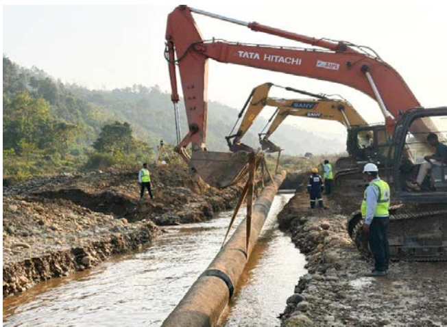
Umiam River Crossing at Chainage 74 Km
