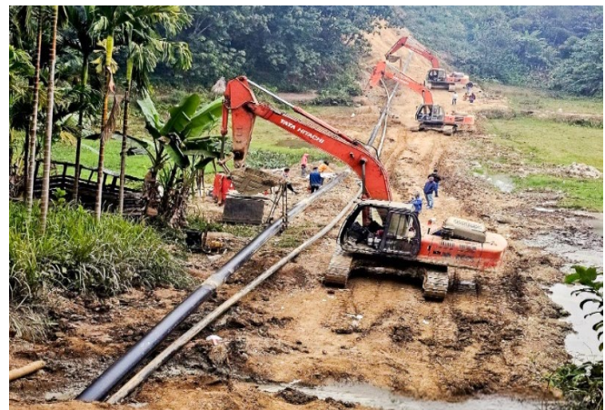
HDD works being carried out at tough terrains along Panisagar-Aizawl Section
